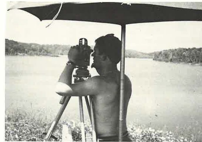
Occupying a part of the section surveyed this summer was Tipsaw Lake, a USFS man-made lake. Extensive horizontal and vertical control was accomplished around the lake. Some plane table mapping was done at the bathing beach site.
