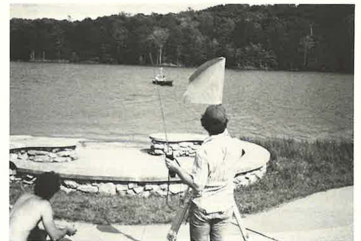
A hydrographic survey was completed of a part of Tipsaw Lake with the aid of a USFS 16-ft. boat and a Purdue Geosciences Department fathometer. The Schneider Engineering Co. of Indianapolis also loaned a second fathometer and boat. Thanks to Luther Condre and the Schneiders.
