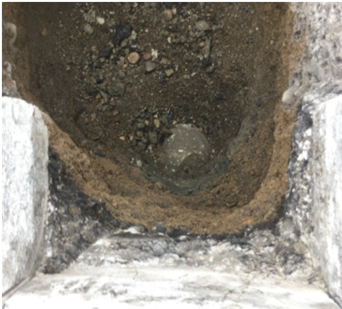
Resting 31 inches below 96th Street in Marion County is a 7-inch by 7-inch quarter corner stone sought by Norman Hiselman, PS and Jim Swift, PS, at a location agreeing with the findings of a 1963 Weihe Engineers survey. (Photo provided by Jim Swift)
