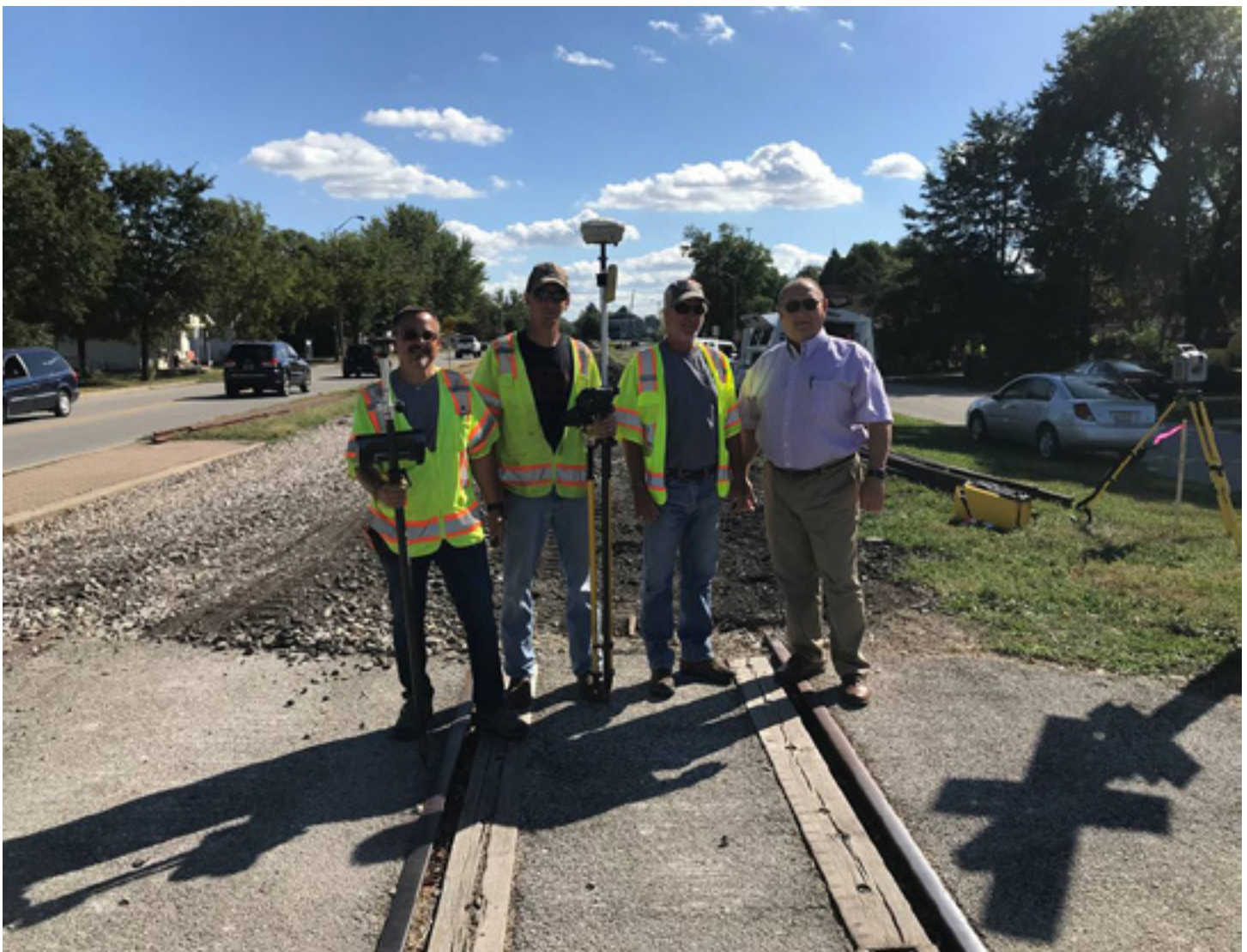
Hamilton County Surveyor Kent Ward (right) and Surveyor's Office crew members (from left) survey manager Brian Rayl, section corner technician Bob King and survey technician Steve Fesmire stand at what's left of the Plum Street crossing in Noblesville, several days after rails and crossies were removed along the former Nickel Plate Railroad line. Ward's crews got ahead of track-removal teams when work began Aug. 16, collecting 600 points to document the centerline between the rails from Noblesville south to the Hamilton-Marion County boundary. (Photo submitted by Todd Whisman)
