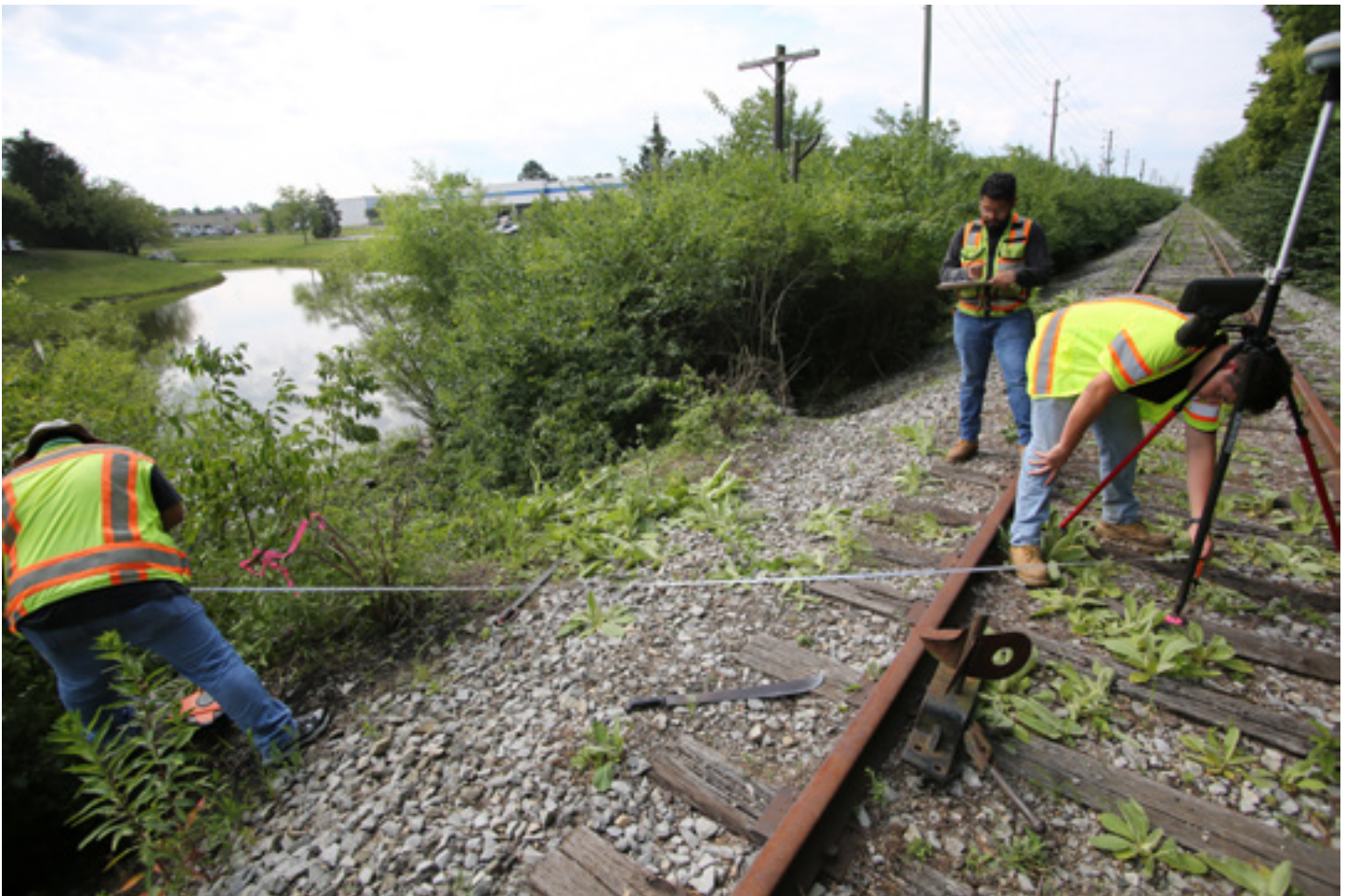
A crew from the Marion County Surveyor's Office measures a distance to a tie along the former Nickel Plate Railroad tracks between 86th and 96th streets. From left are crew chief Robert Pangelinan and surveying technicians Joshua Lindo and Kevin Herrin. The rails and cross ties, which have since been removed, will be replaced by a paved pedestrian trail. (Photos submitted by Ethan Evans)
