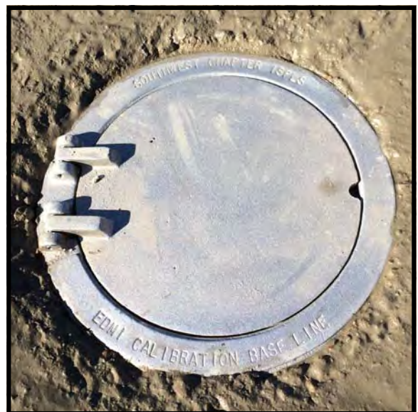
A 5" Berntsen monument lid provides access to the markers approximately 9" below grade. This was done to protect the mark from mowing maintenance and farm equipment.
