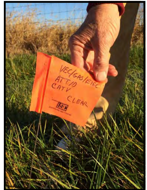
A utility locator's flag gives the all clear for digging.
