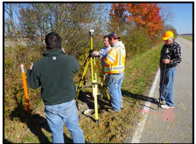
L. to R.: Calvin Cash, Greg Kissel, Matt Badger and Gale Badger prepare for an observation with the Trimble R10 GNSS over one of the marks.
