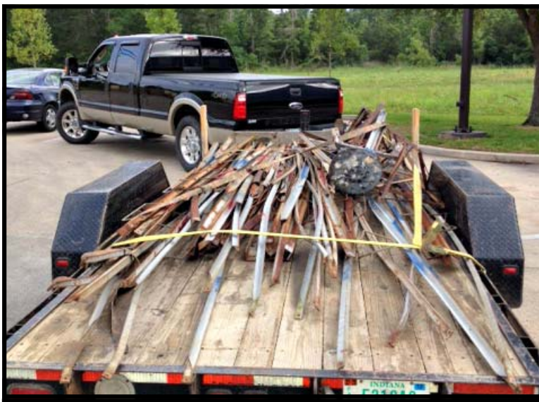
Pieces of a 64-foot Bilby Steel Tower for Triangulation are strapped on a flatbed trailer, ready to begin an 800-mile journey to Indiana from the tower's former site on a Louisiana island. Surveyors Historical Society members plan to reassemble the framework at the Town Park in Osgood, the hometown of the tower's inventor, Jasper Sherman Bilby. (Photo provided by Jeff French)
