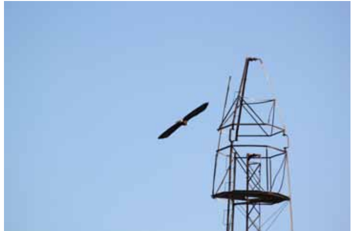
A bald eagle leaves its perch atop the Bilby Steel Tower in the Salvador/Timken Wildlife Management Area. The inner and outer structures are visible in this view.
