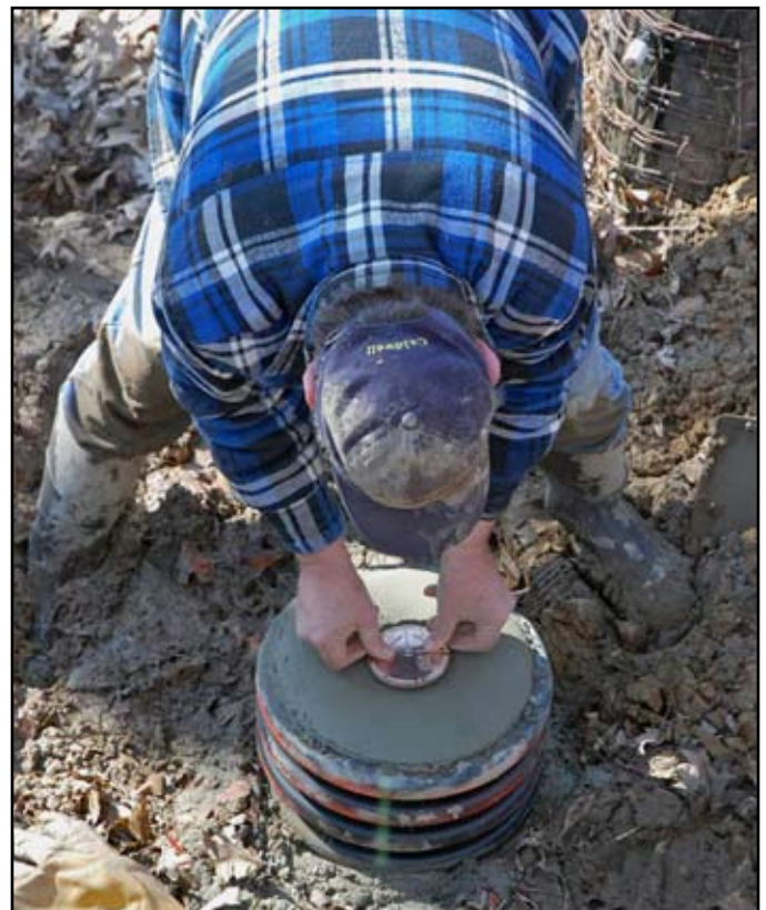
Norman Caldwell, Recording Secretary of the Indiana-Michigan State Line Committee, on April 3, 2008 is shown very carefully pressing the 4" bronze cap into the wet concrete to remonument the northeast corner of the State of Indiana. Located immediately below the concrete-encased monument is a subsurface 4" bronze cap with the same markings set atop a 3" diameter pipe 12 inches in length. Image is courtesy of Duane Brown, P.E., L.S.)
